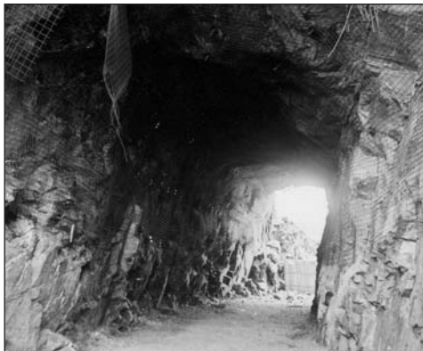
Needle's Eye Tunnel Looking West
